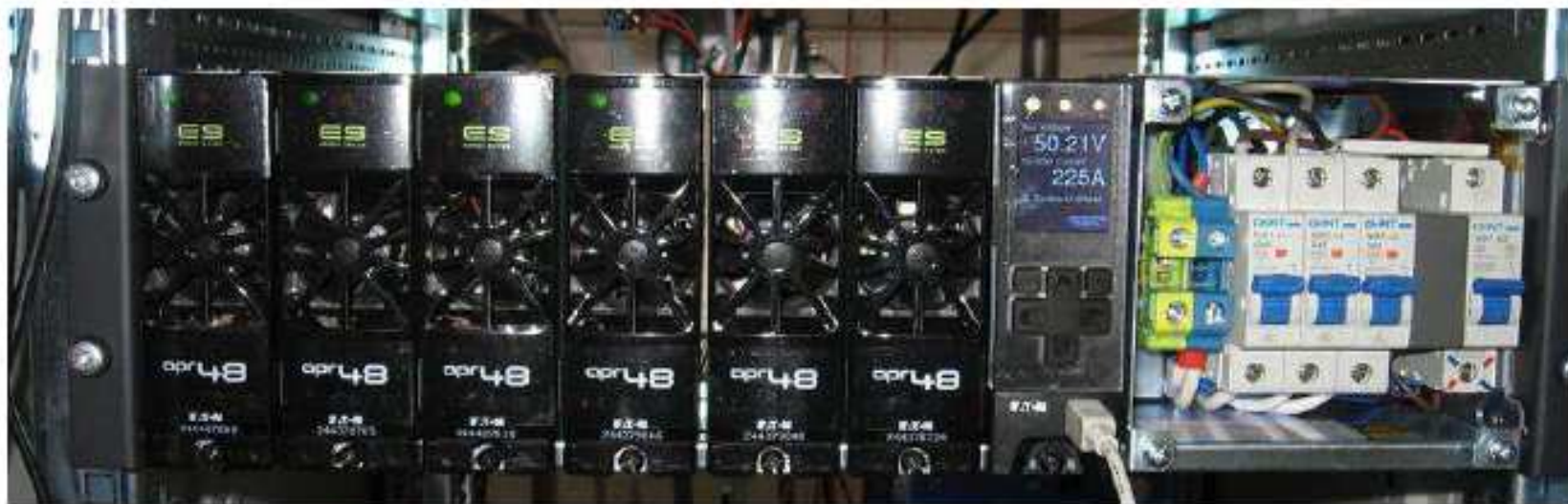
High efficiency (96%) 220 V ac / 50 V dc power converters
